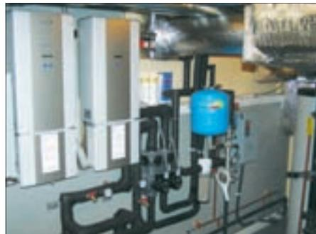
KACO Solar PV inverters create AC power used by the ground-water source heat pump system.
