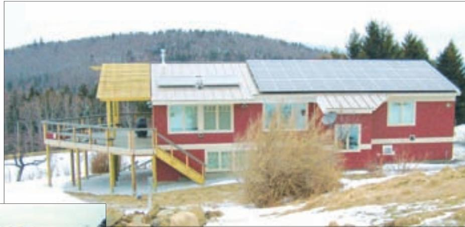
South rooftop PV solar system is calculated to provide greater annual summer production due to low roof pitch. Two additional flat plate solar collectors provide hot water to occupants with any surplus contributing to space heating needs.
